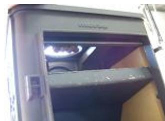
13. Finally move the boiler into position and fix using the washers and locking nuts provided
